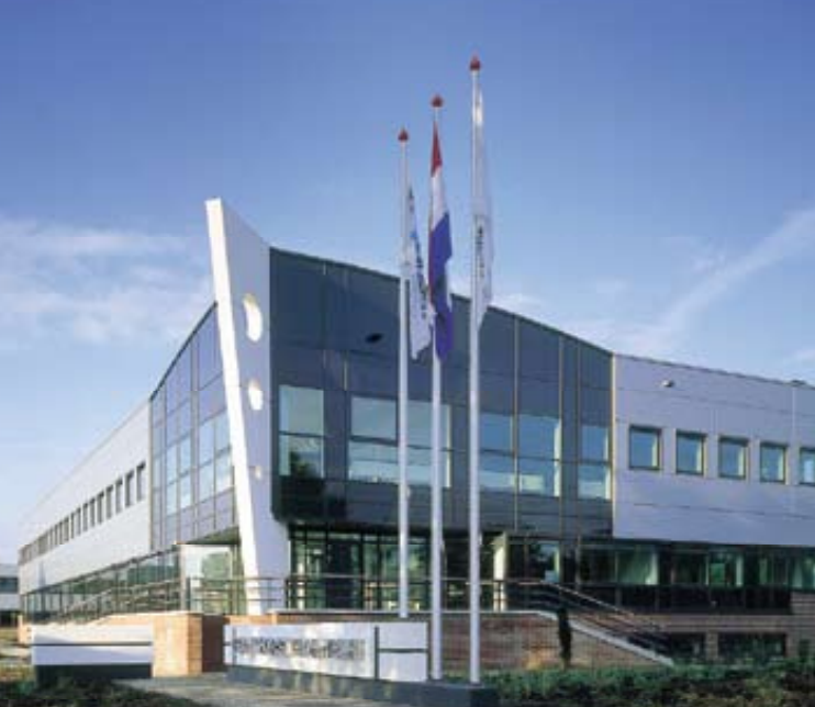
Bronkhorst High-Tech headquarters, The Netherlands
